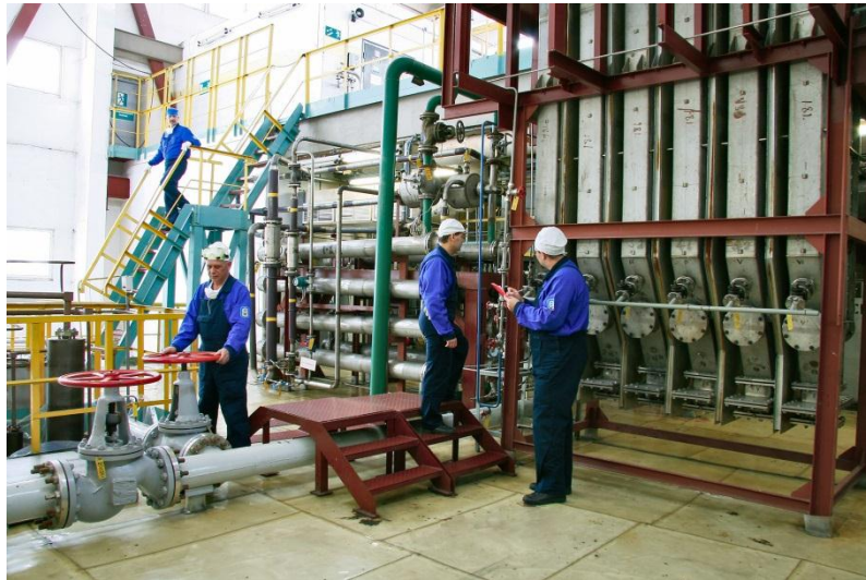
Burning stove of solid radioactive waste
