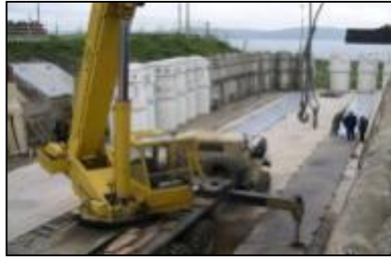
Cranage and lifting equipment
