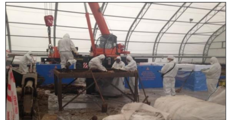
Decommissioning of the radwaste storage facility
