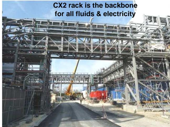
CX2 rack is the backbone for all fluids & electricity
